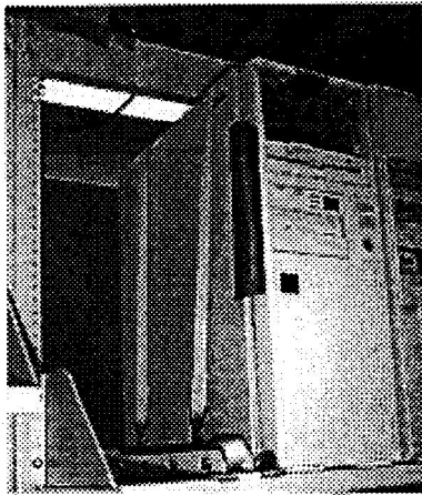
Figure 5 - attachments to CPU on LAN rack
